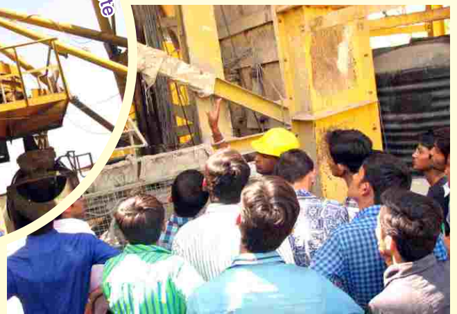
Plant official explaining the process of Concreting
